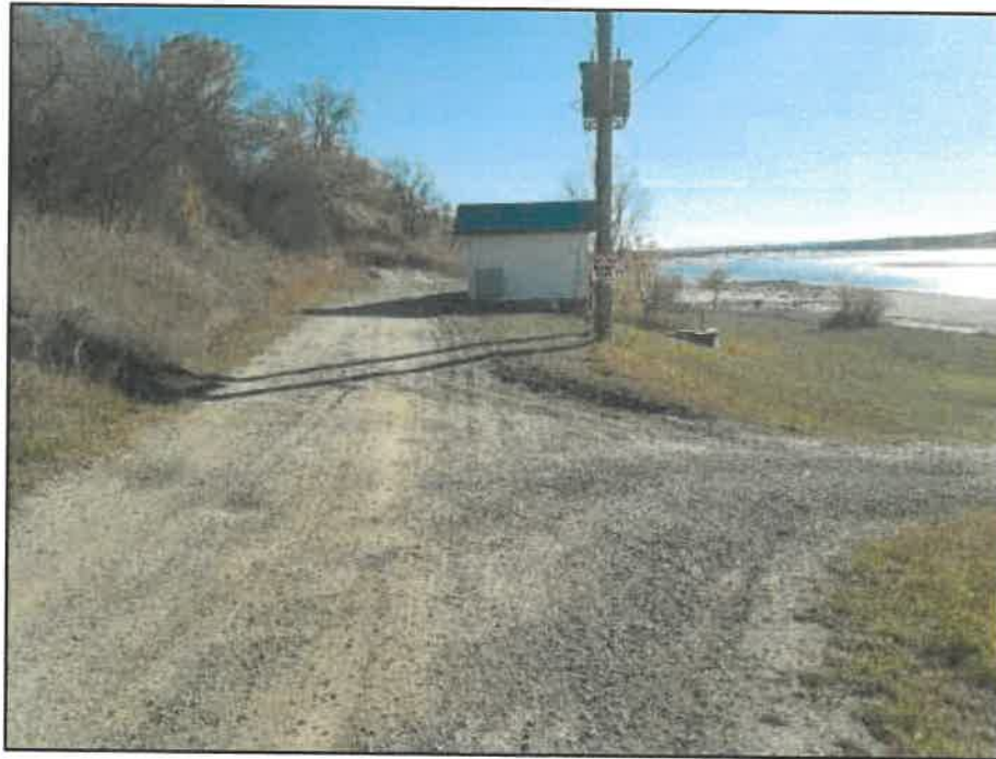
PHOTOGRAPH NO. 18533-03: Existing raw water pumphouse at toe of east slope. Power line was tight.
