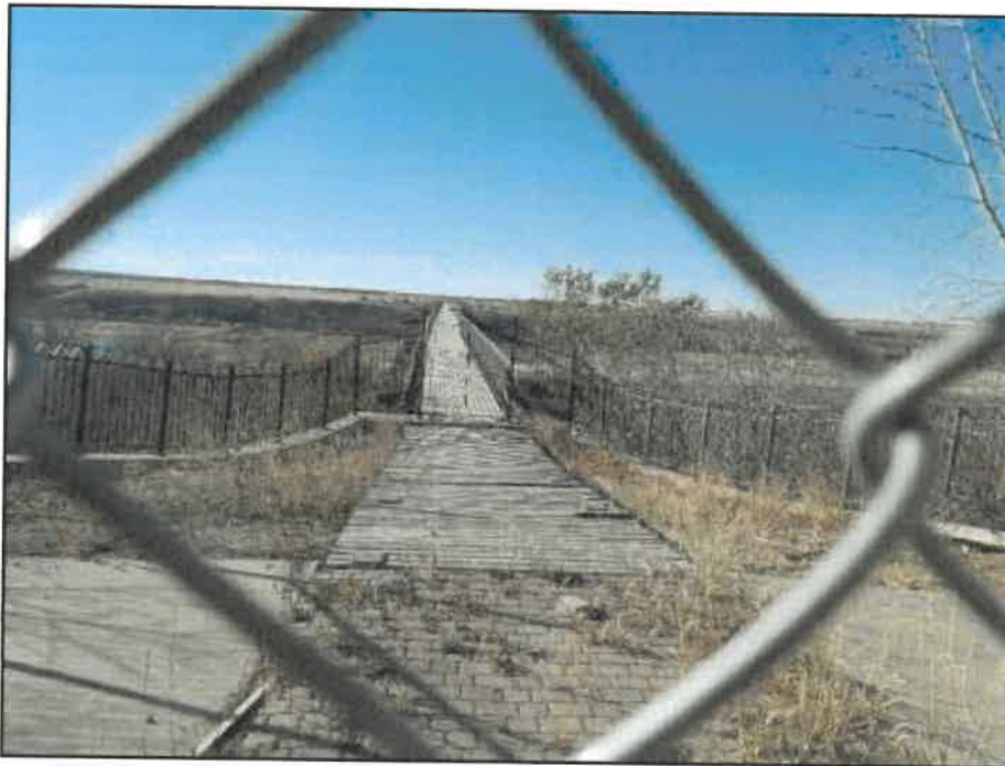
PHOTOGRAPH NO. 18533-08: Looking west from east abutment of rail bridge.
